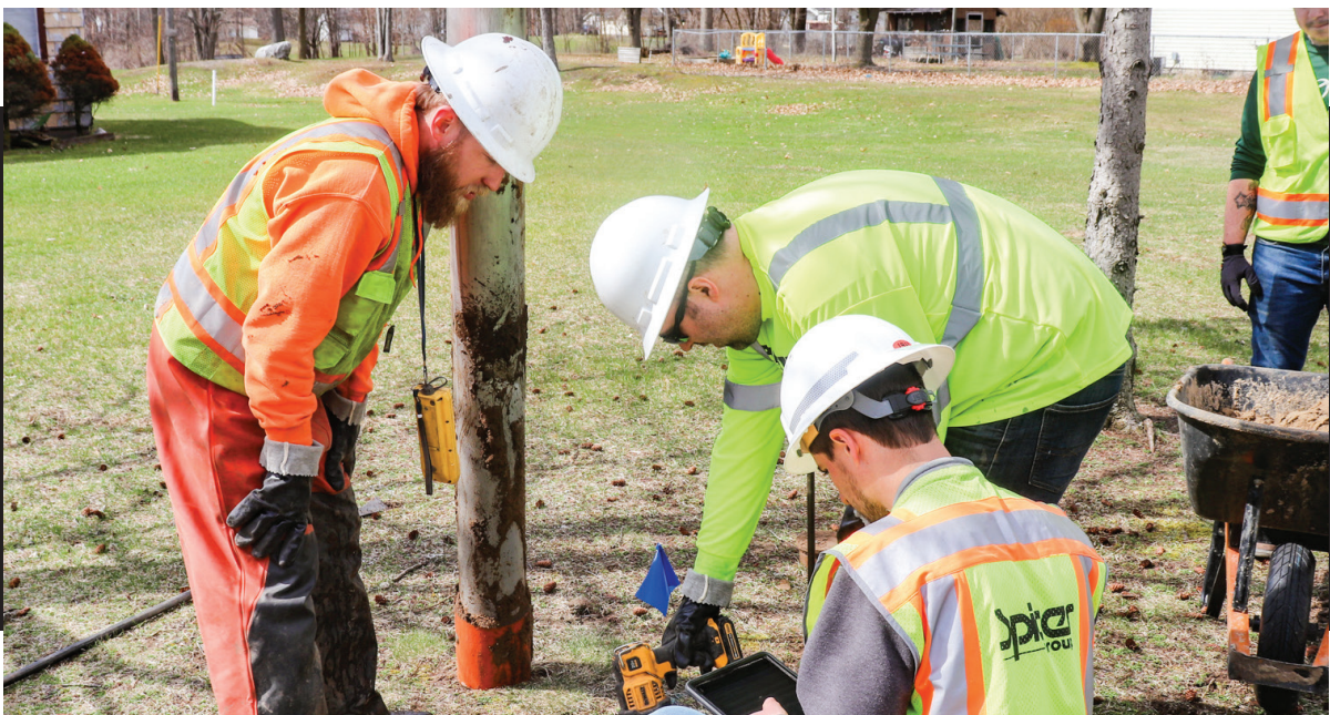
Spicer Group Inc. engineer Neil Noack working with Underground Infrastructure Services to hydroexcavate, identify, and record the materials of water services in the Village of St. Charles.
