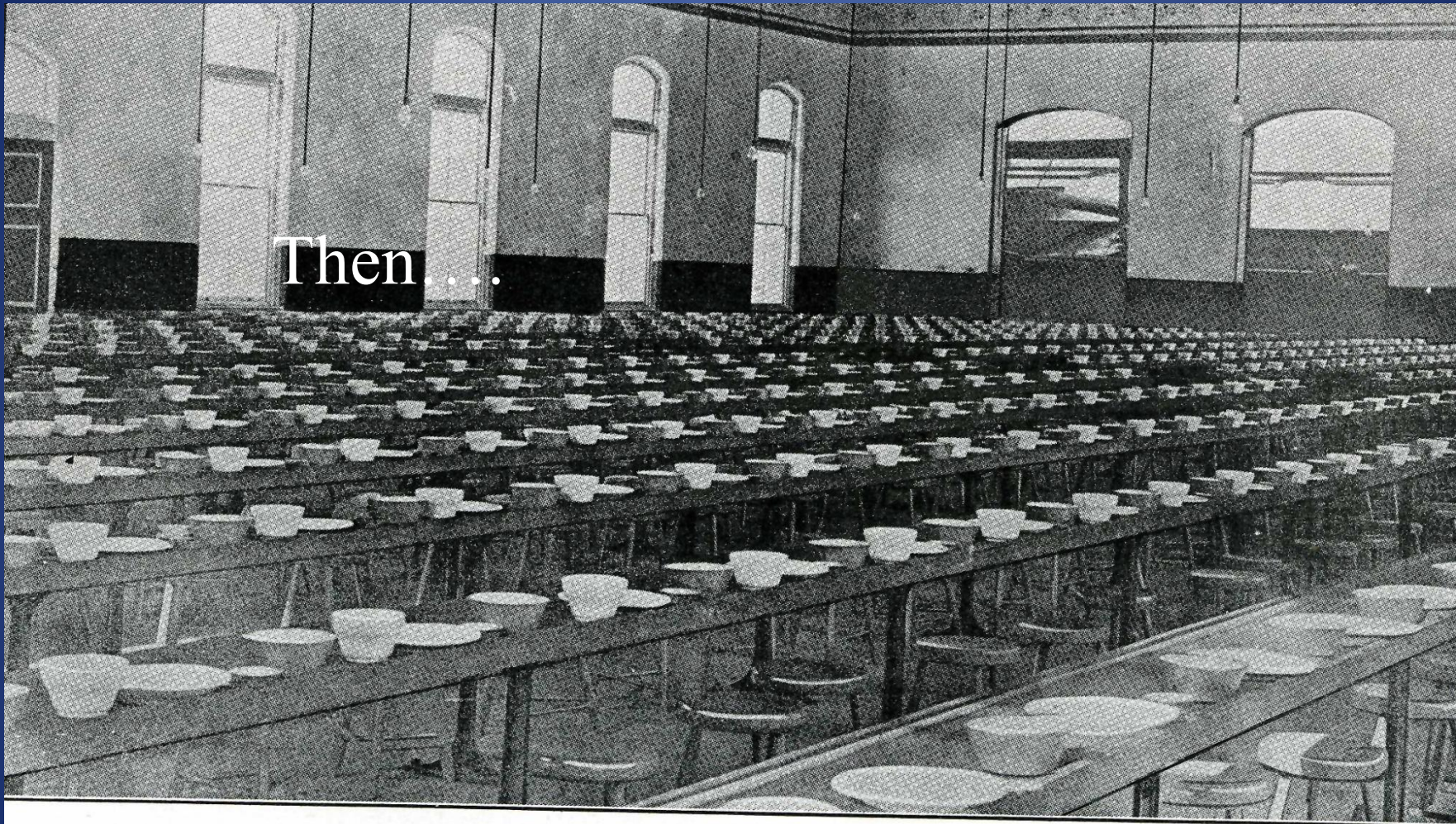
INTERIOR OF DINING ROOM—MICHIGAN STATE PRISON
